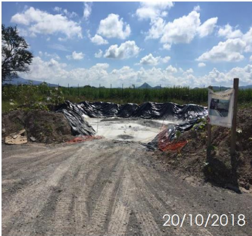
2.3.1.1 Concrete wash-out.
