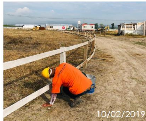
2.1.2.8. The area of gardens was preserved from construction activities with a temporary fence, made from recycled wood, painted with paint crafted on-site made from lime and salt.
