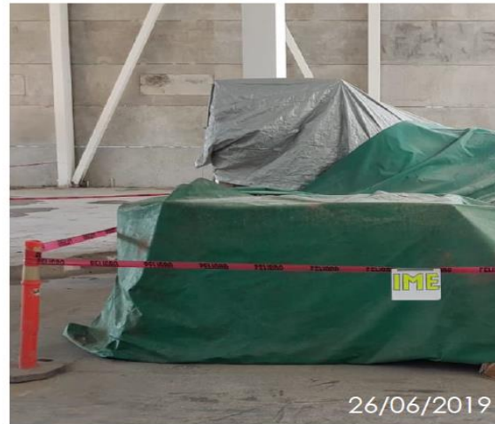
2.3.3 Protection of sensitive to moisture materials.
