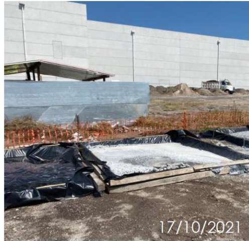
2.3.1.1 Concrete wash-out
